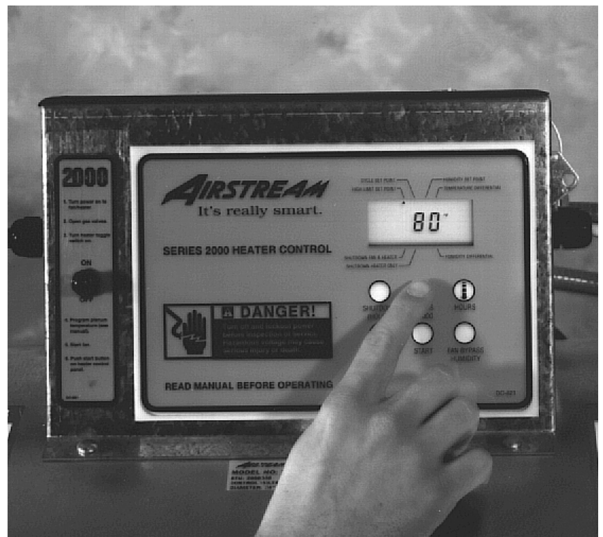
Programming the high-limit set point.
